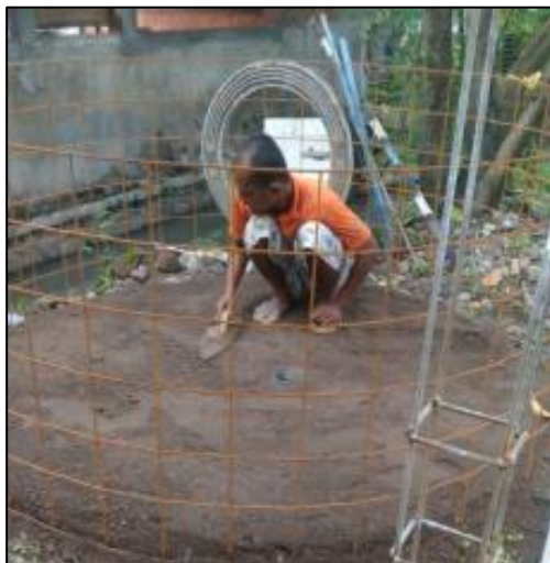
Figure 3. Pool assembly (source: team documentation)
