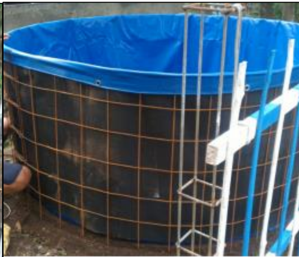
Figure 4. Tarpaulin pond construction (source: team documentation)
